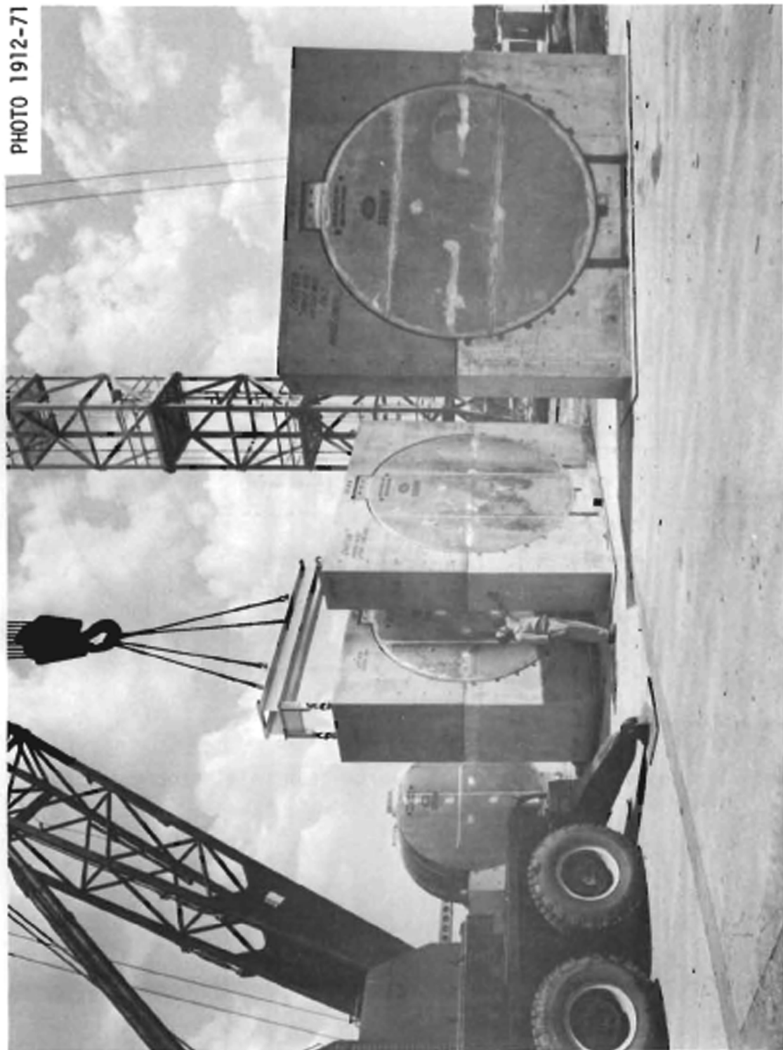
Fig. 2. Photograph of the sodium tanks. The concrete collar had not as yet been attached to the 5-ft. tank in the background.
